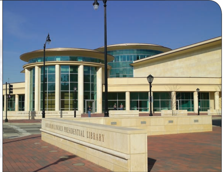
One hundred VAV controllers are tied to a series of sensors and AHUs to maintain the collection of priceless artifacts at the Abraham Lincoln Presidential Library in Springfield, IL.
